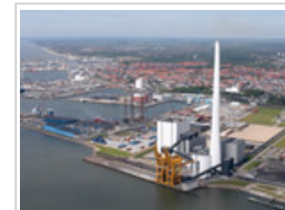
The Esbjerg Power Station, a CO 2 capture site in Denmark. Source: DONG Energy
