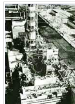
The destroyed reactor Source: Chernobyl Forum
