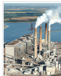
The Gibson coal power plant, a good example of a large stationary source. Source: John Blair, valleywatch.net [see http://valleywatch.net ]
